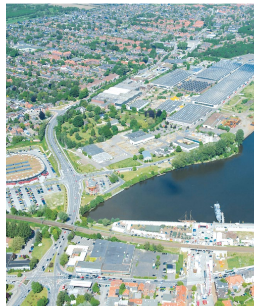
ACO Group headquarters in Rendsburg/Büdelsdorf
